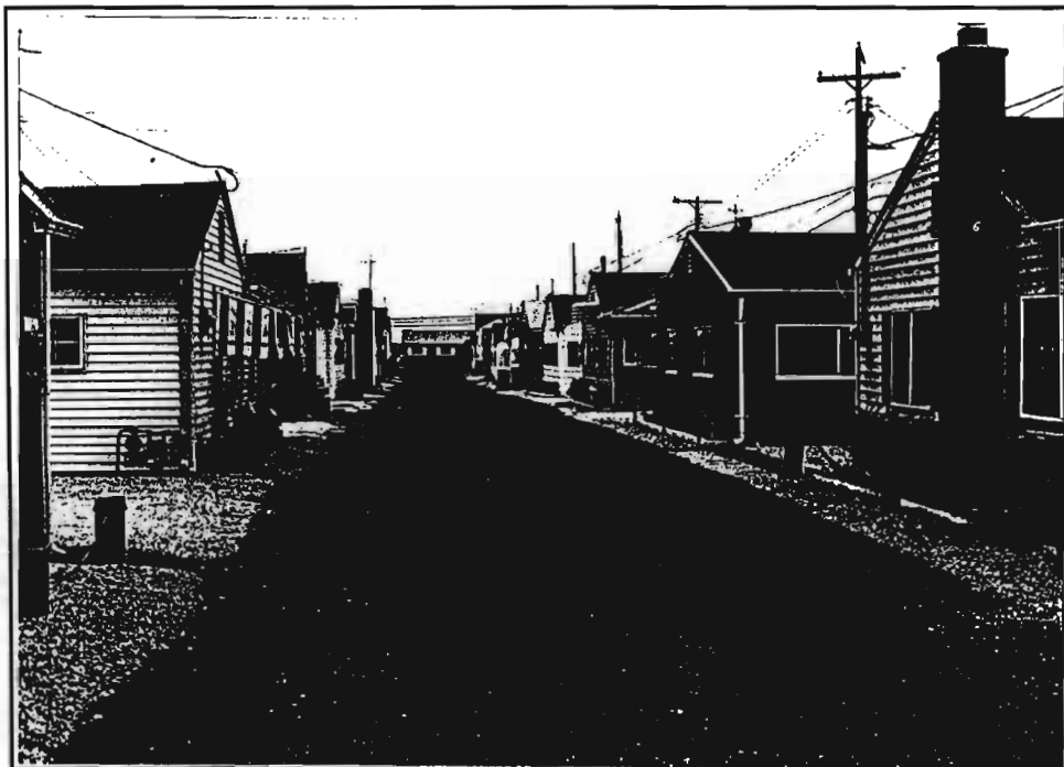
West on West Shell Way from NJ Rte. 35 northbound, Ocean Beach Unit 2 Dover Township, Ocean County, NJ Dover Township Tax Map Block 1105.11 & 1105.12
