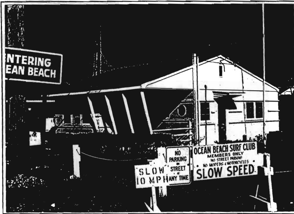
35 East Surf Way, Ocean Beach Unit 1 Dover Township, Ocean County, NJ Dover Township Tax Map Block 1102.02, Lot 2 Representative resource - west and south facades
