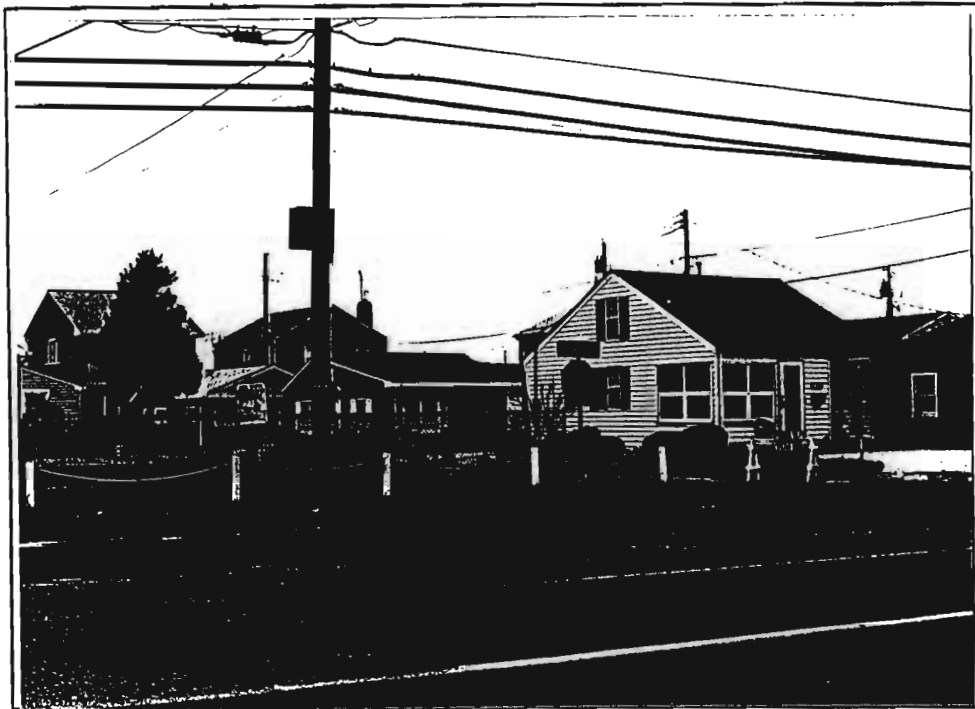
West side of NJ Rte. 35 northbound at West Beach Way, Ocean Beach Unit 1 Dover Township, Ocean County, NJ Dover Township Tax Map Block 1101.05 & 1105.06
