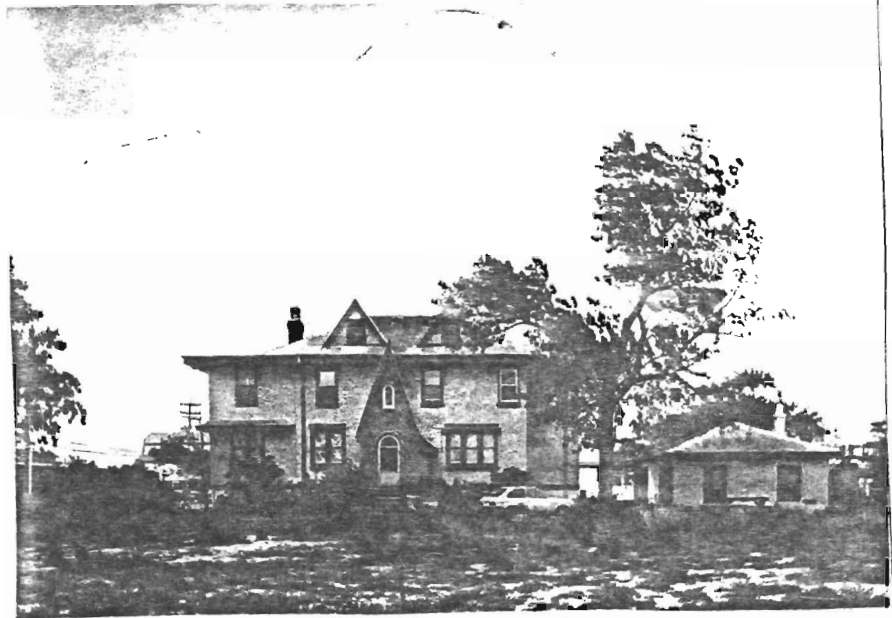
West Point Island House / Washington Avenue and Bay Boulevard
