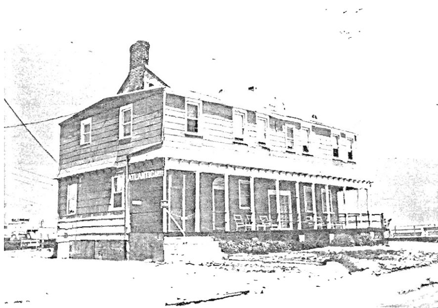
Atlantic Apartments / 1 Atlantic Avenue
