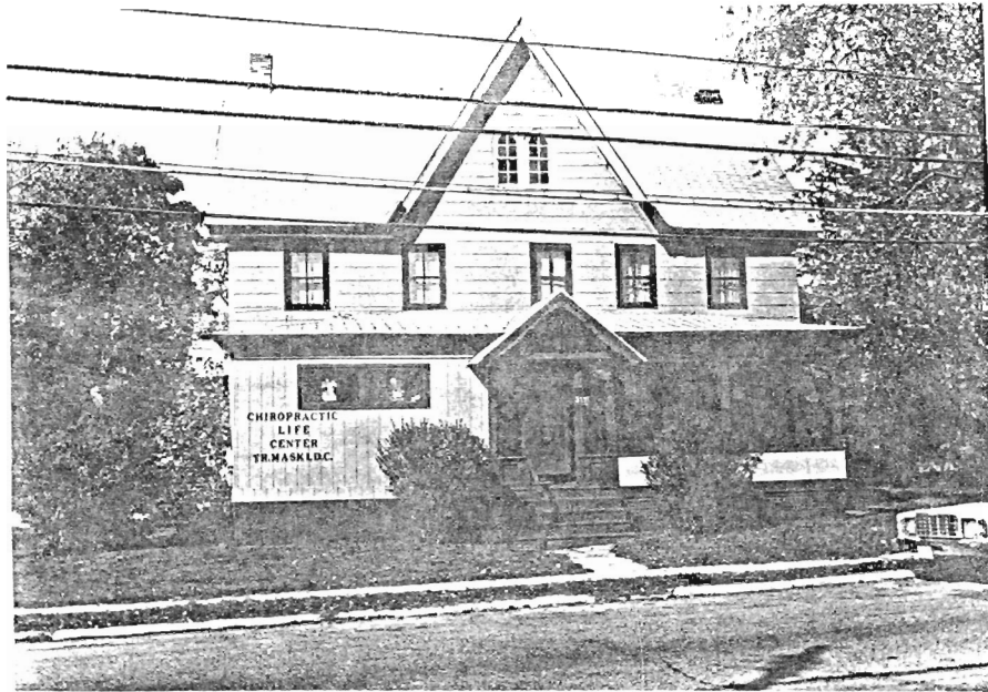
Austin House / 317 Main Street
