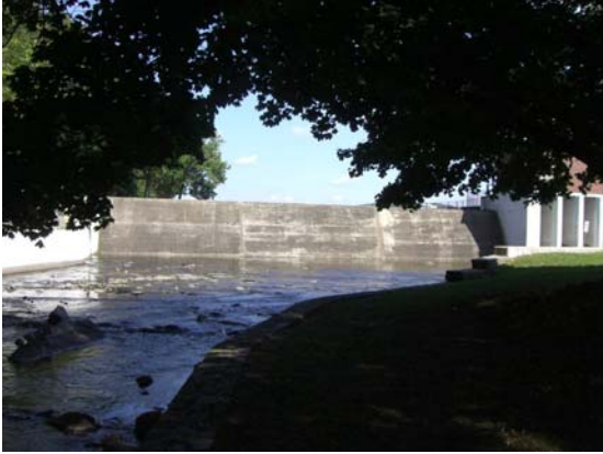
Lake Hopatcong Dam
