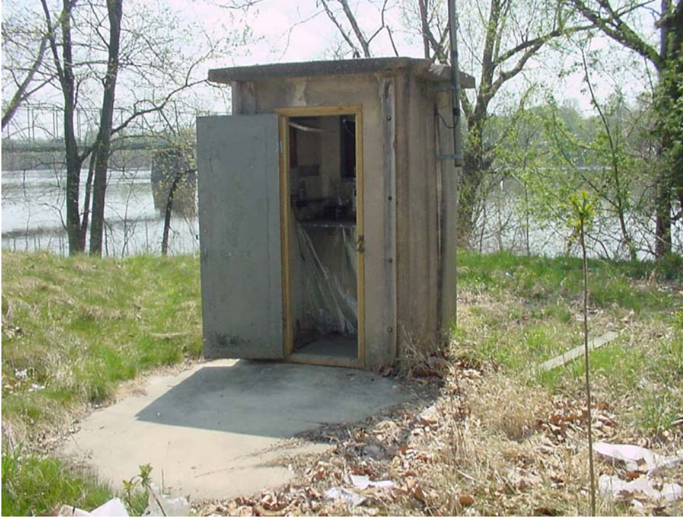
Photo 1: View of the pre-hardened USGS gage at the Delaware River Trenton (01463500).
