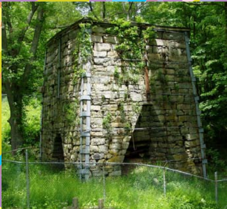
Furnace at Wawayanda State Park, Sussex County
