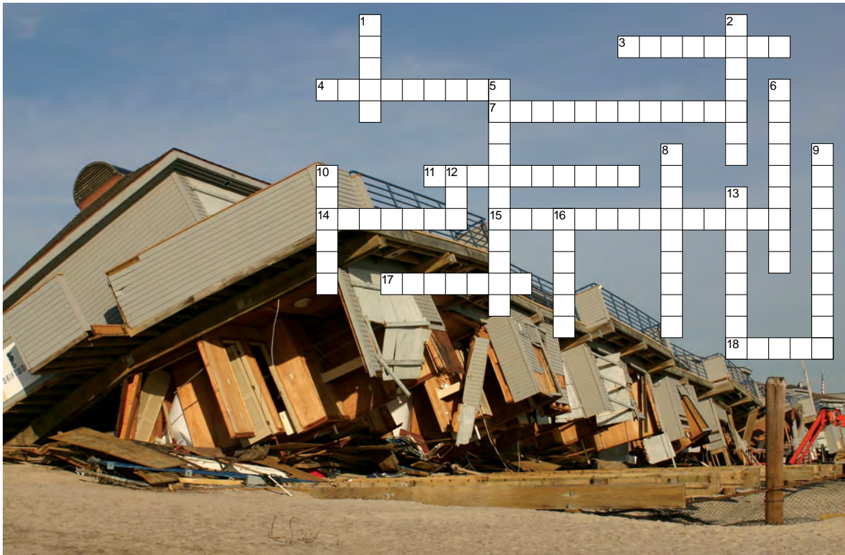
Structure pushed off its foundation by Hurricane Sandy storm surge, Sea Bright Boro, Monmouth County. Photo by Z. Allen-Lafayette
