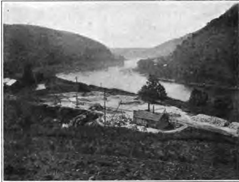
Fig. 1. View through Weygadt, on the Delaware River, above Phillipsburg.
