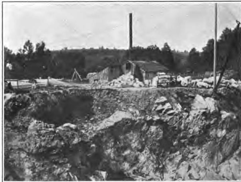
Fig. 2. Warne's Serpentine Quarry, near Phillipsburg.
