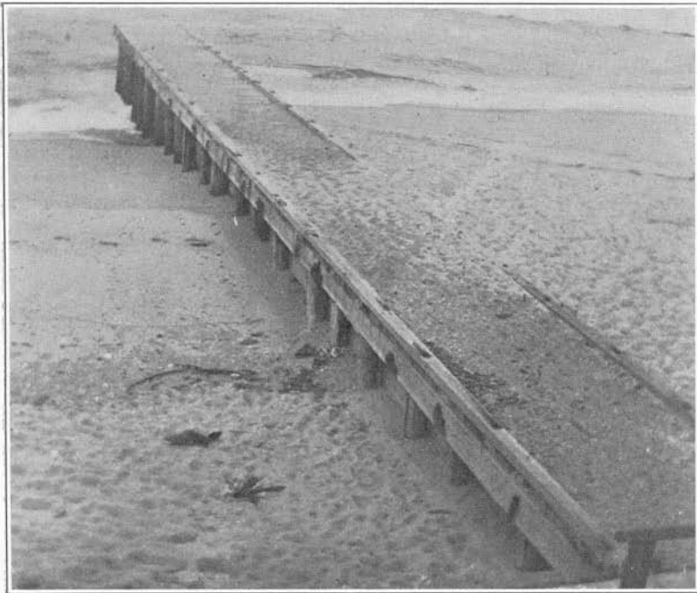
Fig. 1. Spur jetty or groyne at Long Branch.
