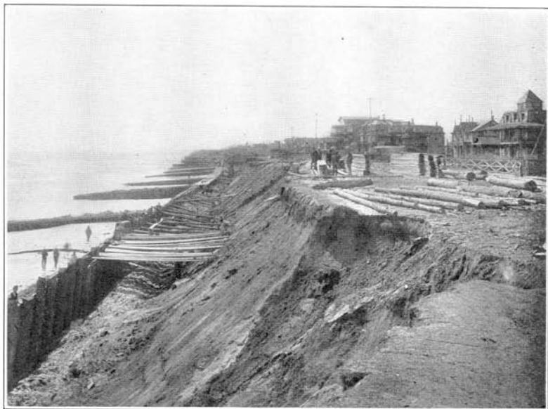
Jetties and bulkhead at Long Branch.
