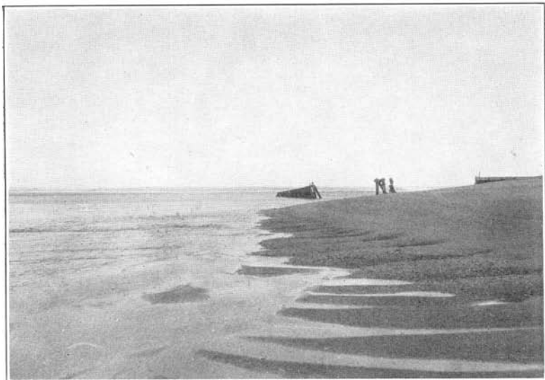
Fig. 1. Deposit of sand at the Belmar bulkhead June 6, 1905.
