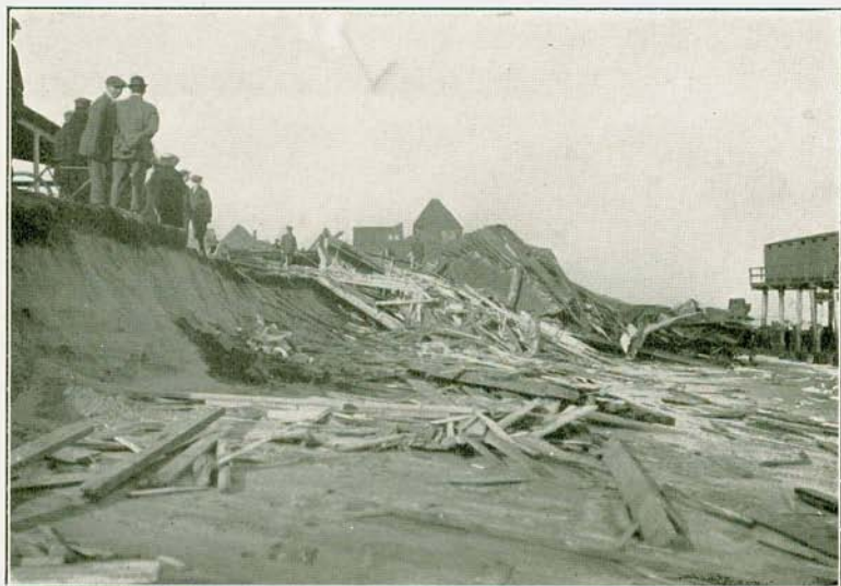
PLATE III, FIG. 1.—Storm cliff cut in seaward edge of bar at Sea Bright, showing houses demolished by undermining, and unharmed bath-houses on pilings.
