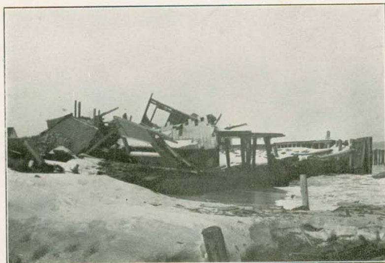
PLATE II, FIG. 2.—Same house as in Plate II, completely destroyed by the waves. Remnants of hulkhead and outlying lines of pilings seen at right.
