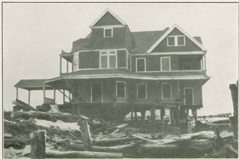
PLATE II, FIG. 1.—Same house as in Plate II, almost completely undermined by the waves. Wave-cut cliff seen at left.
