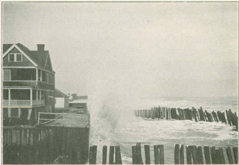
PLATE I, FIG. 1.—House at Monmouth Beach protected by bulkhead and outlying rows of piling. See Plate II, Fig. 2, and Plate III, Fig. 1 and 2.
