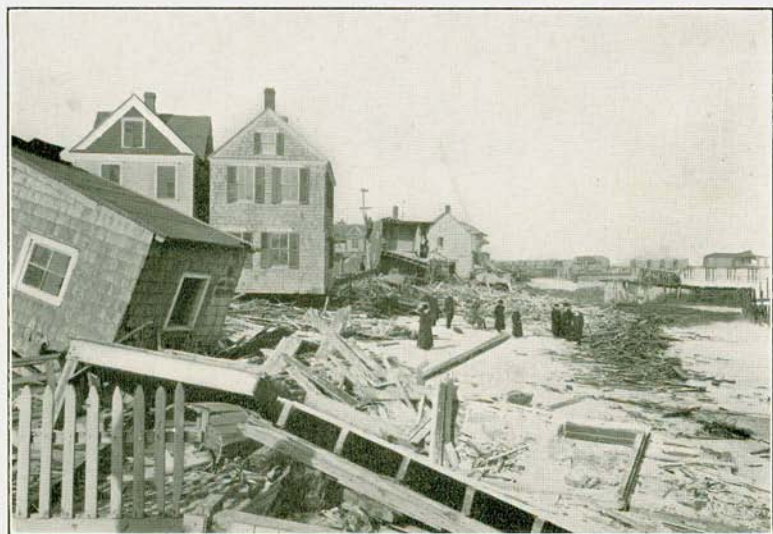
PLATE III, FIG. 2.—Scene on the shore at Sea Bright after the New Year's Storm, showing undermined houses, and piles of wreckage on beach.
