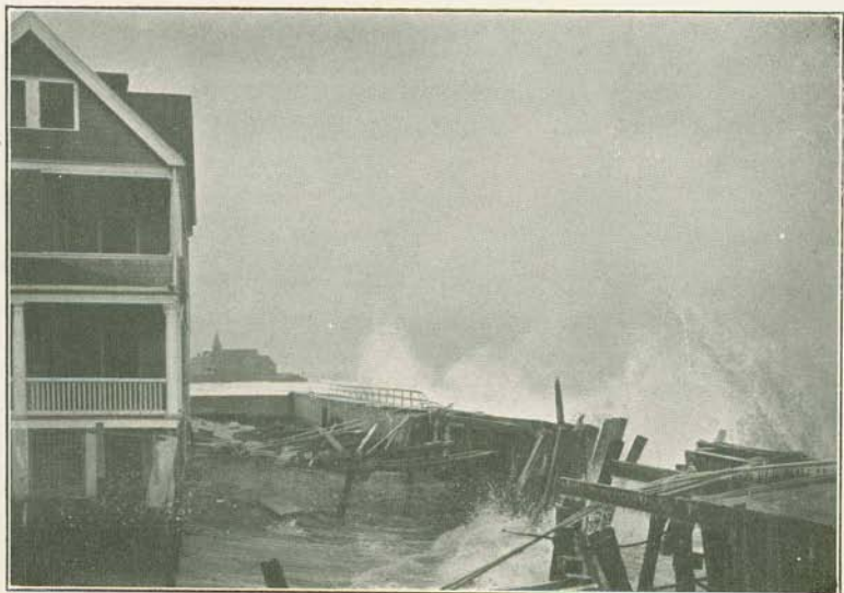
PLATE I, FIG. 2.—Same house as in Plate II, Fig. 1, showing breaching of protecting bulkhead. Undermining of one corner of house just beginning. NEW JERSEY GEOLOGICAL SURVEY
