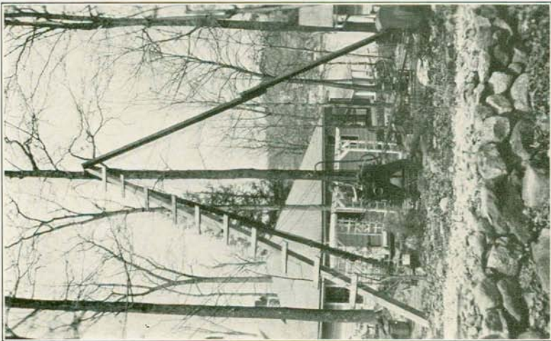
(a) A type of machine used for drilling in hard rock. Cutting action is produced by the use of small steel shot under the rotated bit.
