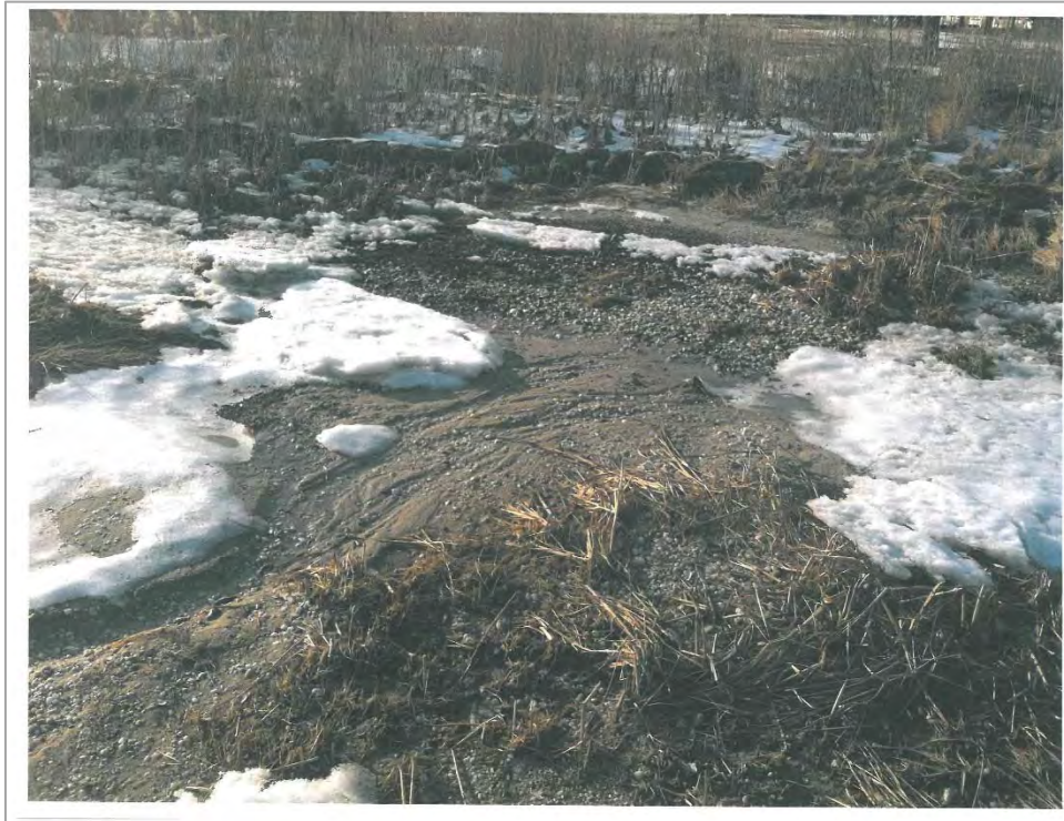
Figure 10: Area 2 – sandy wash out area
