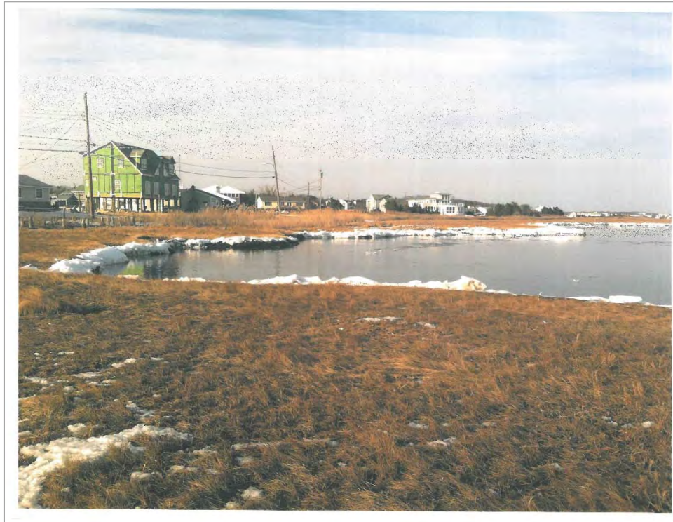
Figure 7: Area 2 – eroded shoreline, facing south
