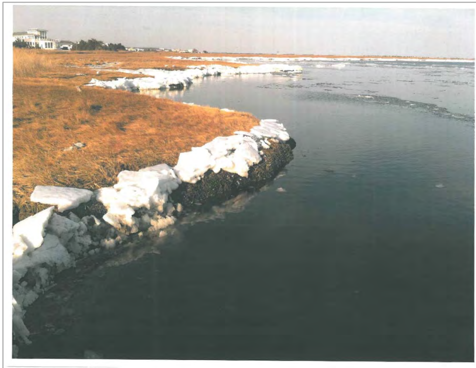
Figure 8: Area 2 – eroded shoreline, facing south
