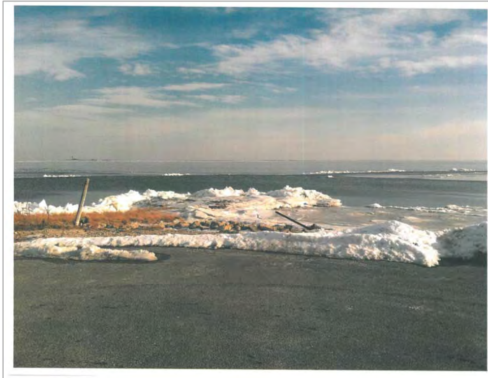
Figure 5: Area 1 – View south towards the Bay
