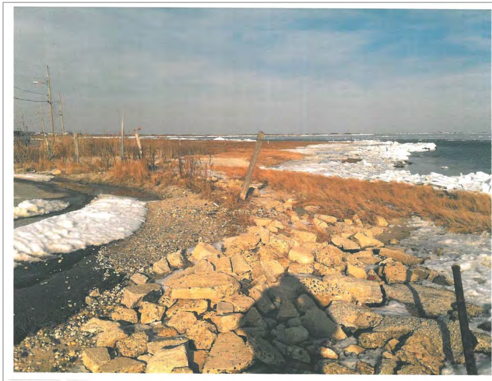
Figure 4: Area 1 – concrete debris at the Iowa Court Cul-de-Sac
