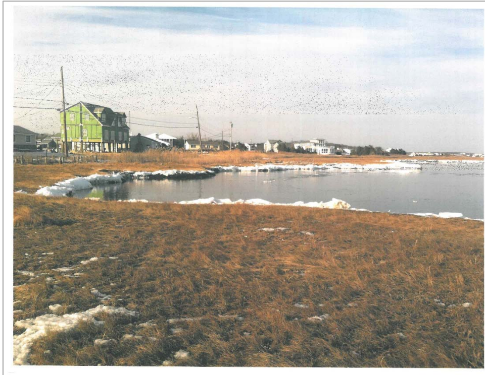
Figure 7: Area 2 – eroded shoreline, facing south
