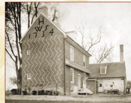
West elevation featuring herringbone brick pattern
