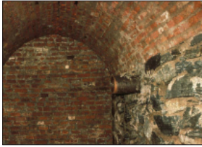
Inside the Petty's Run Culvert
