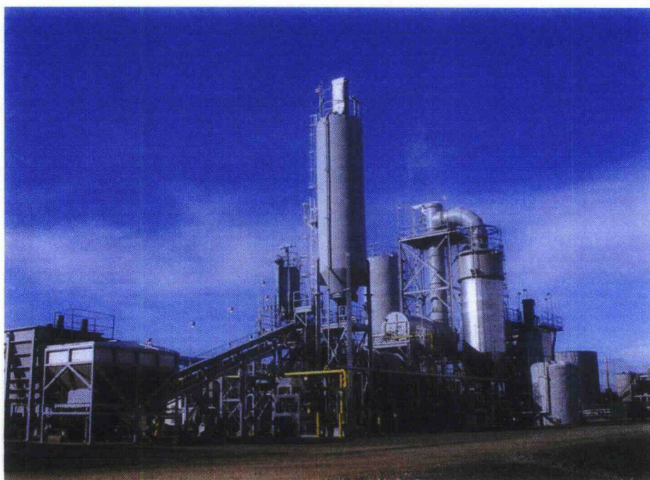
Figure 3. The Cement-Lock Demonstration Plant from the Northeast
