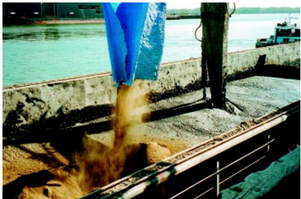
Figure 7-4. Solidification/stabilization processing of dredged material from NY/NJ Harbor. Portland Cement and fly ash are being added through the chute at the left. The column at the right is the drive shaft for a mixer used to homogenize the mixture. The processing is done in the barge used to transport the material for placement at an upland site.
