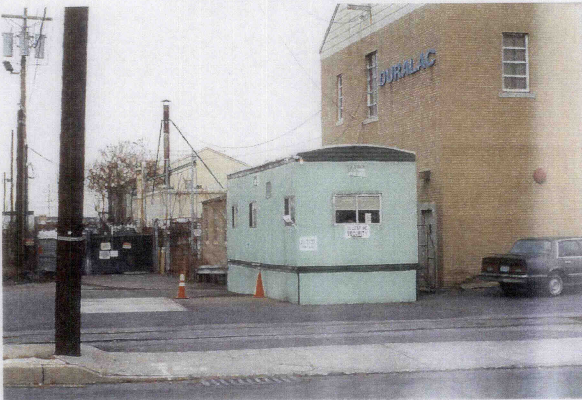
SUBJECT PROPERTY - SECURITY BUILDING
