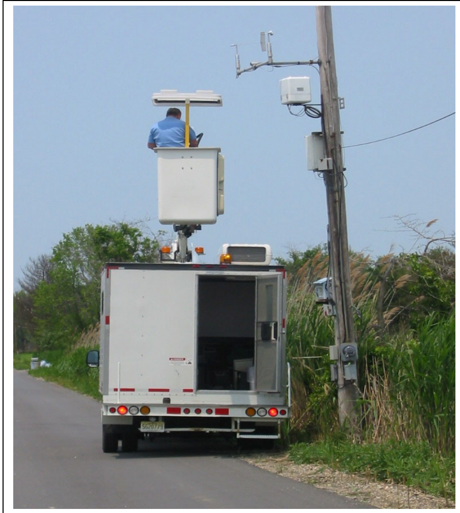
Figure 4: Servicing a CREST Monitoring Station near the Salem / Hope Creek Nuclear Generating Station
