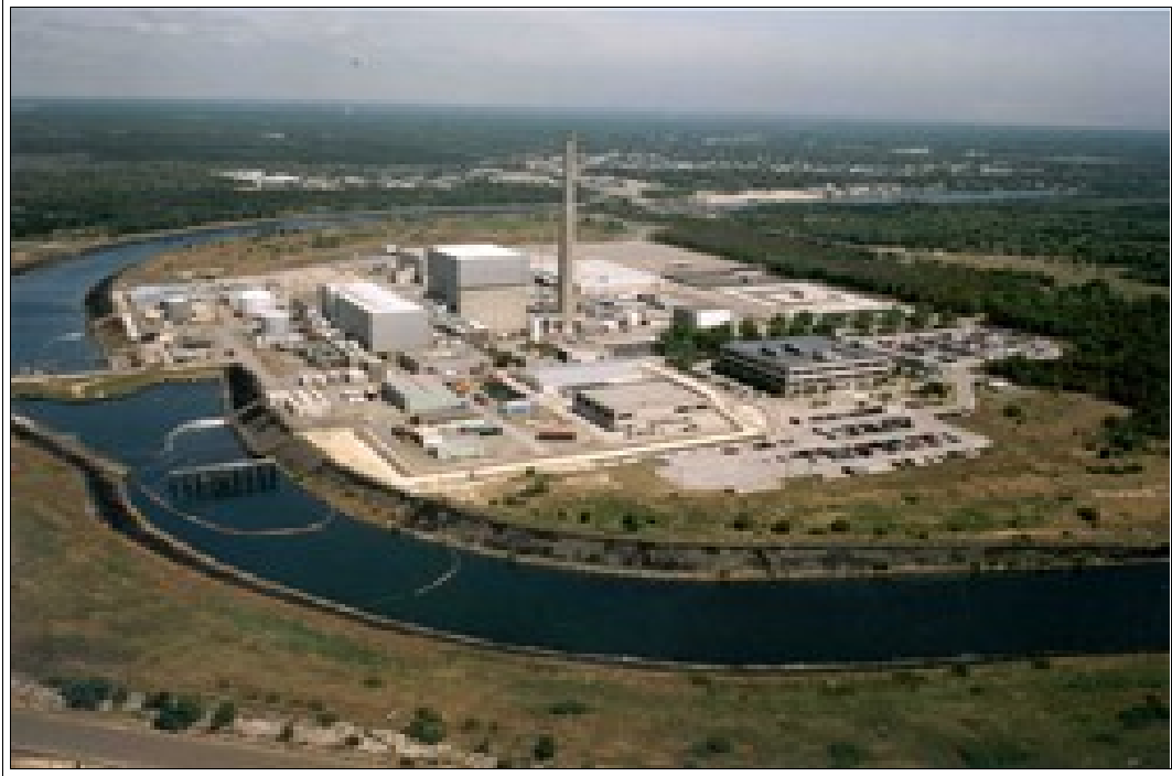
Figure 5 – Oyster Creek Nuclear Generating Station
