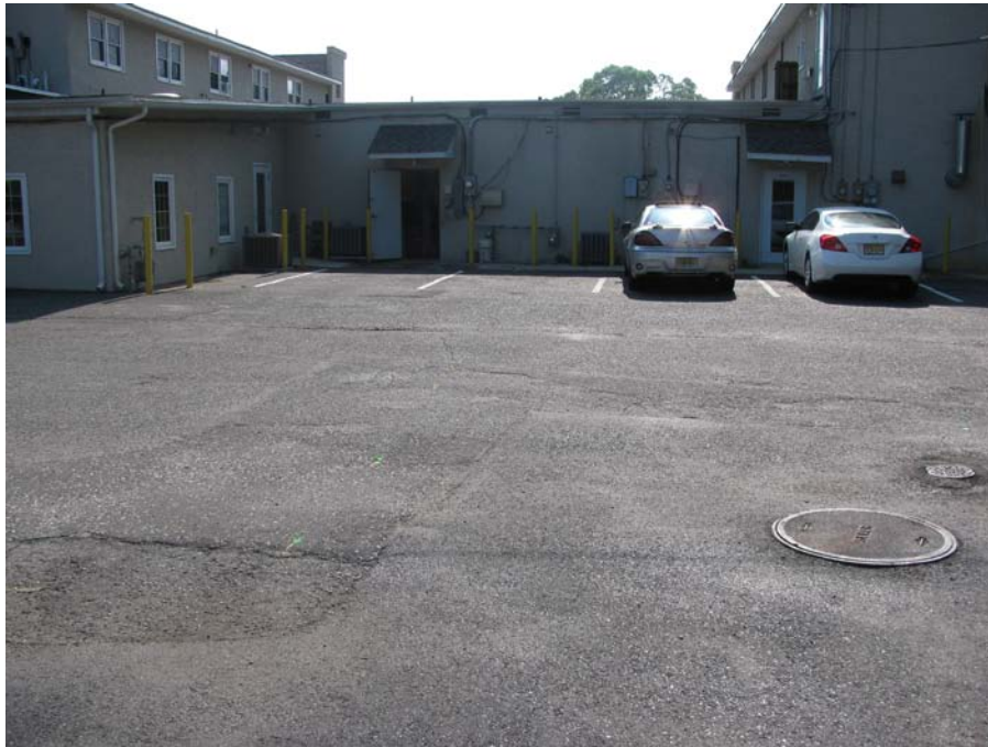
Photograph 3: Facing East, a view of the parking lot and two sanitary manholes; lines run perpendicular to the septic field behind the complex.
