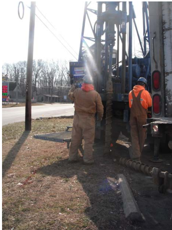
Photograph 7: Close up of Summit Drilling during monitoring well installation; drilling at MW02 (on Site) using a Hollow Stem Auger (HSA).
