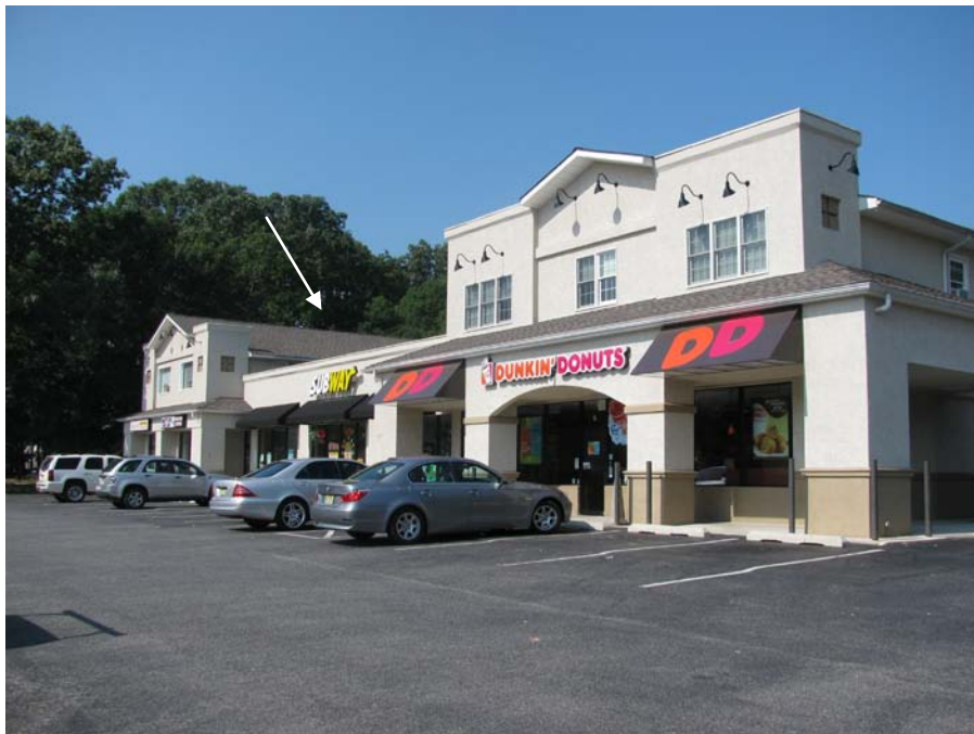
Photograph 5: Looking South at the current commercial complex, note that the Site is currently occupied by Subway, adjacent to Dunkin Donuts.
