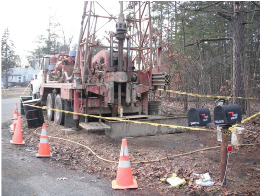
Photograph 10: Close up of Mud Rotary Rig, used to install 3 deep wells (MW13, MW14 and MW07).
