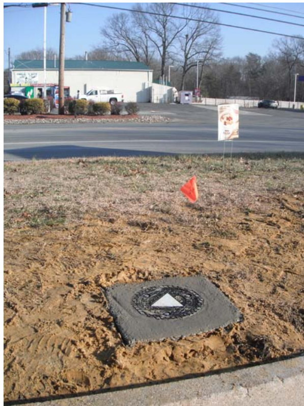
Photograph 9: Completed flushmount well with cement pad (MW02).
