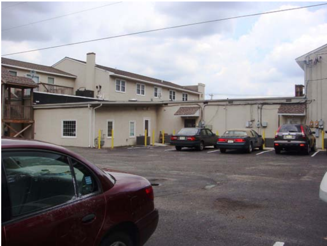
Photograph 2: View of rear of building; looking east.
