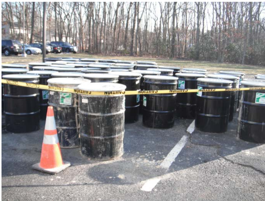
Photograph 11: On-Site drum staging (adjacent to septic field) of non-hazardous soil cuttings and purge water during monitoring well installation.
