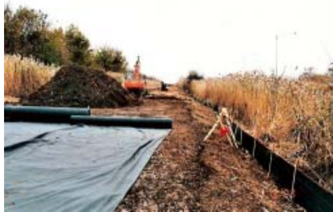
Geotextile Deployment for Roadway
