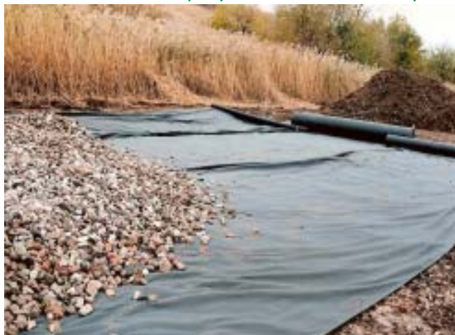
Placing Recycled Concrete on Geotextile
