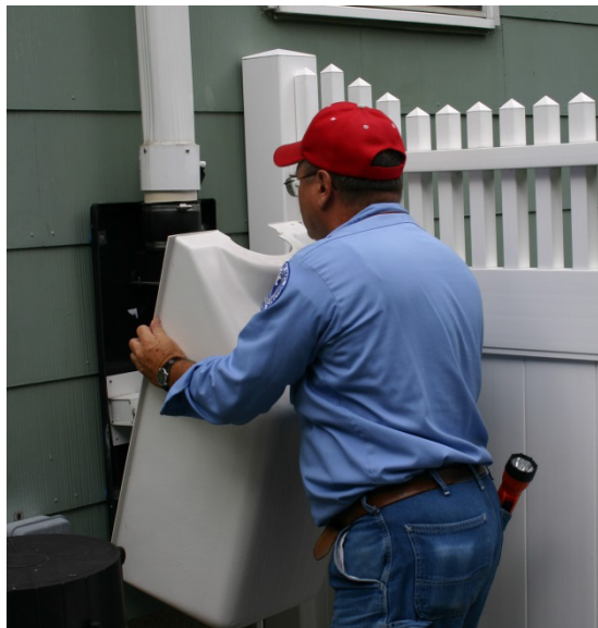
Figure 6-1 Inspection of SSD fan and weatherproof
