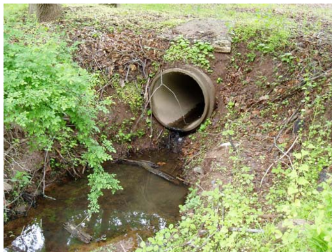
Figure 9. Active storm water outfall in Holland Brook.
