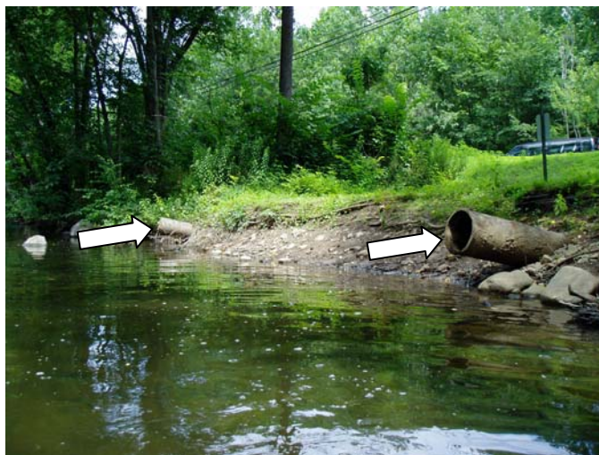
Figure 15. Storm sewer outfalls near the start on the Rockaway River
