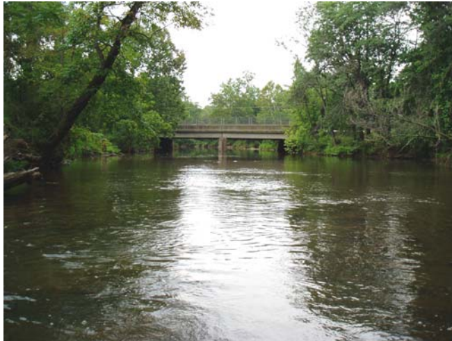
Figure 11. Downstream view showing open canopy and channelization near bridge.
