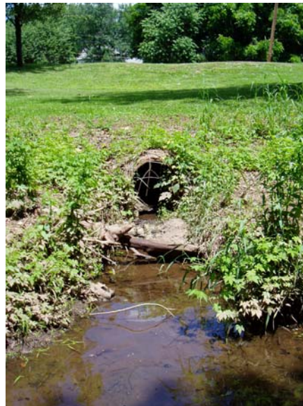
Figure 18. Storm sewer outfall and mowed grass along banks of Peters Brook.
