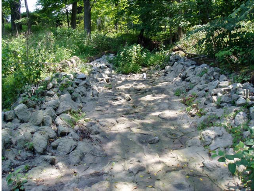
Figure 8. Concrete sluice below several storm water outfalls on the Passaic River
