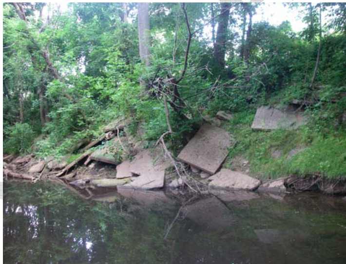
Figure 6. Concrete slabs lining the banks of Royce Brook.
