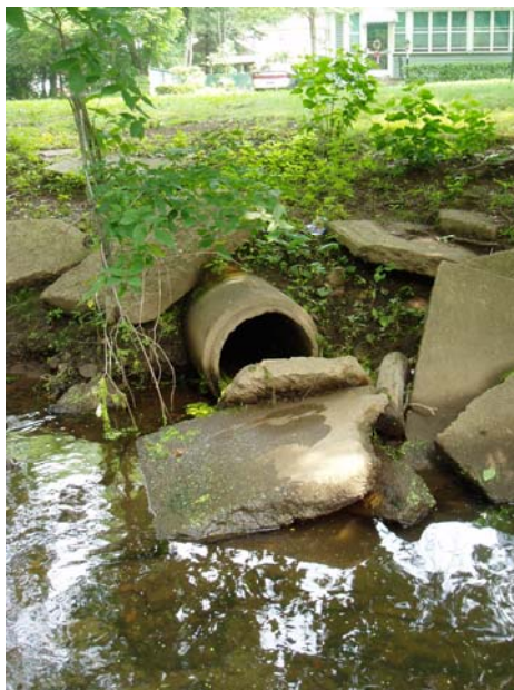
Figure 16. Storm sewer outfall and concrete slabs on Rahway River.
