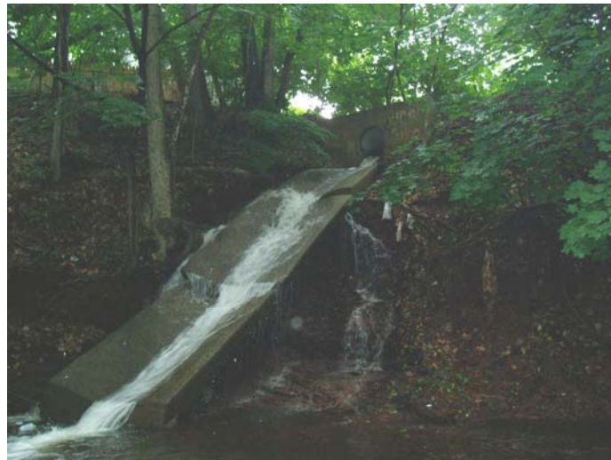
Figure 10. Active storm sewer outfall during storm event at Mile Run.
