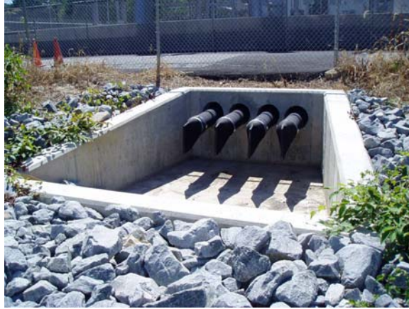
Figure 12. Multiple outfalls on Whippany River.
