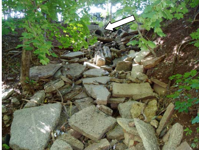
Figure 11. Concrete slabs below large storm sewer outfall on Mile Run.
