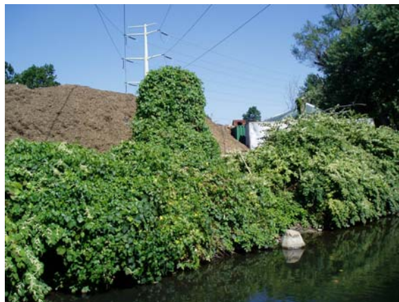
Figure 13. Mulch pile on bank of Whippany River.
