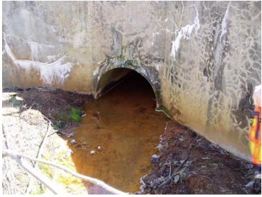
Figure 12. Stormwater outfall pipe at Oakford Lake.
