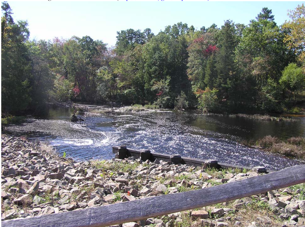
Dam below Batsto Lake, Hammonton, NJ
