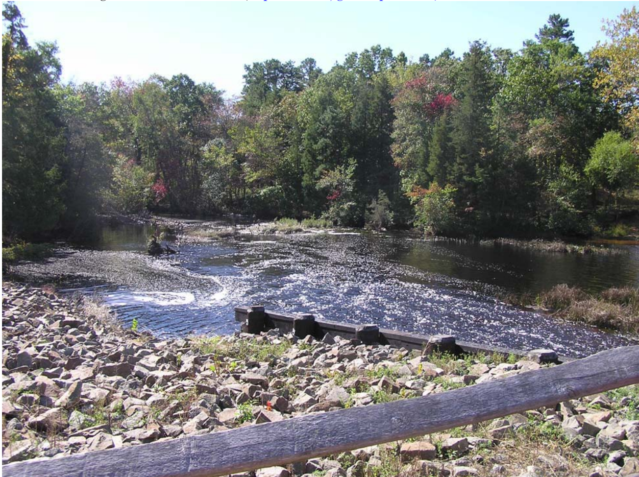
Dam below Batsto Lake, Hammonton, NJ
