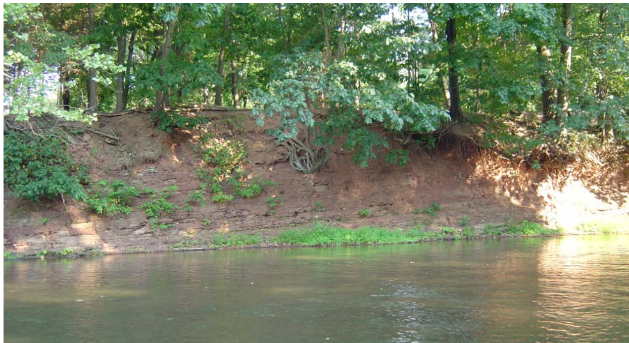
Figure 7: Stream Bank Erosion in North Branch Raritan River
