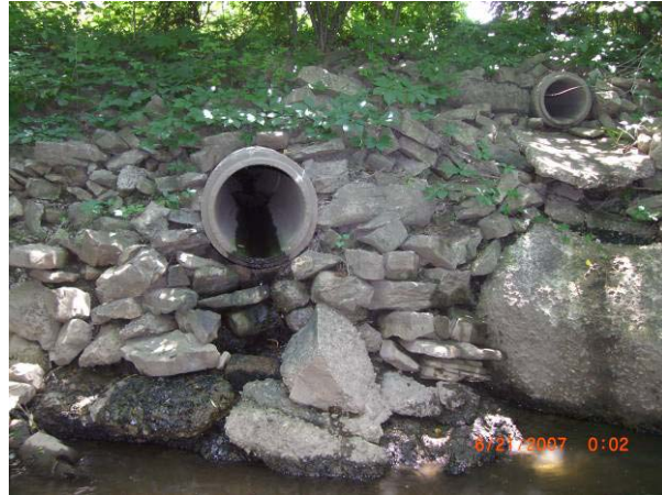
Figure 19. Storm water outfalls on Deepavaal Brook.
