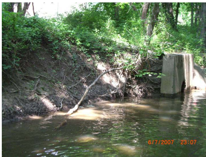
Figure 14. Bank erosion and scouring on Shabakunk Creek.
