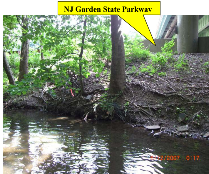
Figure 18. Proximity of NJ Garden State Parkway to Third River.
