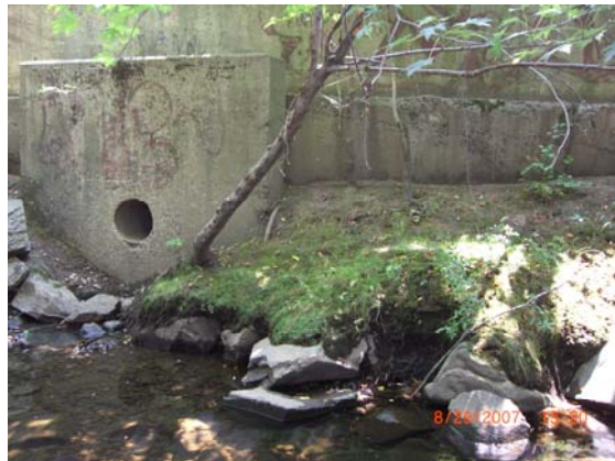
Figure 13. Storm water outfall on Goffle Brook.
