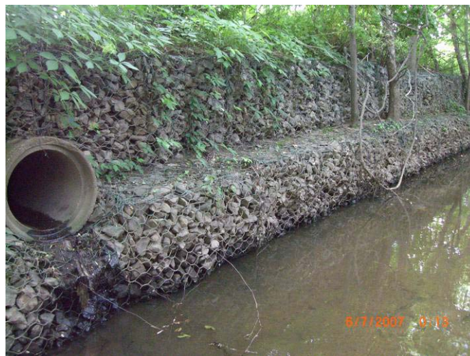
Figure 7. Gabion reinforced bank on Beaver Dam Brook
