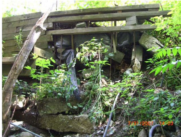
Figure 8. Collapsed retaining wall.
