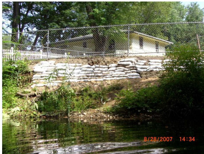
Figure 10. Sandbags used to reinforce bank.
