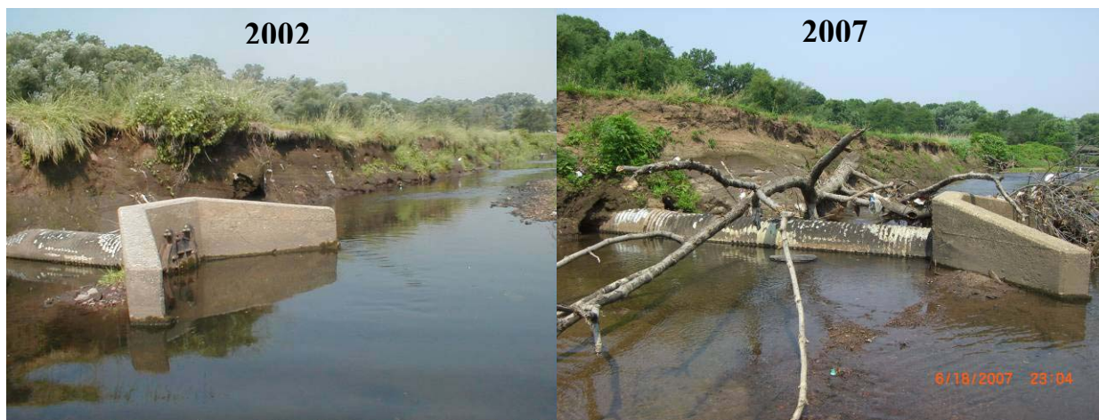
Figure 16. Severe bank erosion on Elizabeth River
