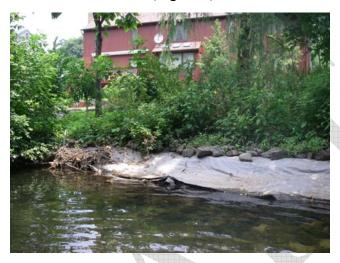
Figure 8. Fabric used to control bank erosion on Saddle River.
