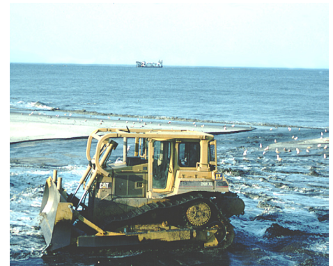
Figure 2. Bulldozer building a protective beach using sands pumped from an offshore sand source. The hydraulic dredge is on the horizon.
