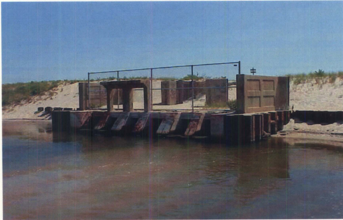
Figure 1.1. The downstream weir structure for Wreck Pond. Photograph courtesy of Mr. C. Tucker, NJDEP.
