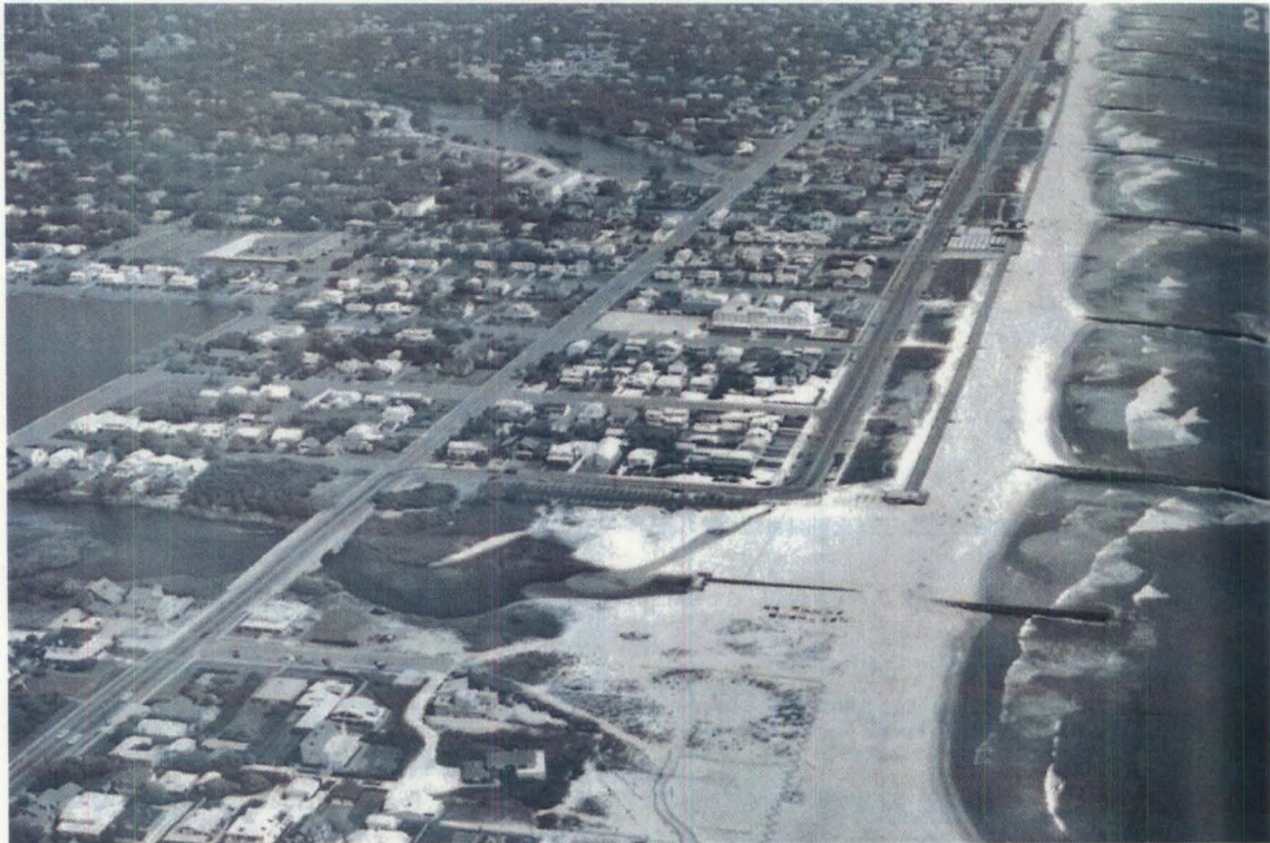
Figure 5.1. June 1987 aerial photograph of Spring Lake, NJ. Existing Wreck Pond outfall pipe is located at the bottom of the photograph.
