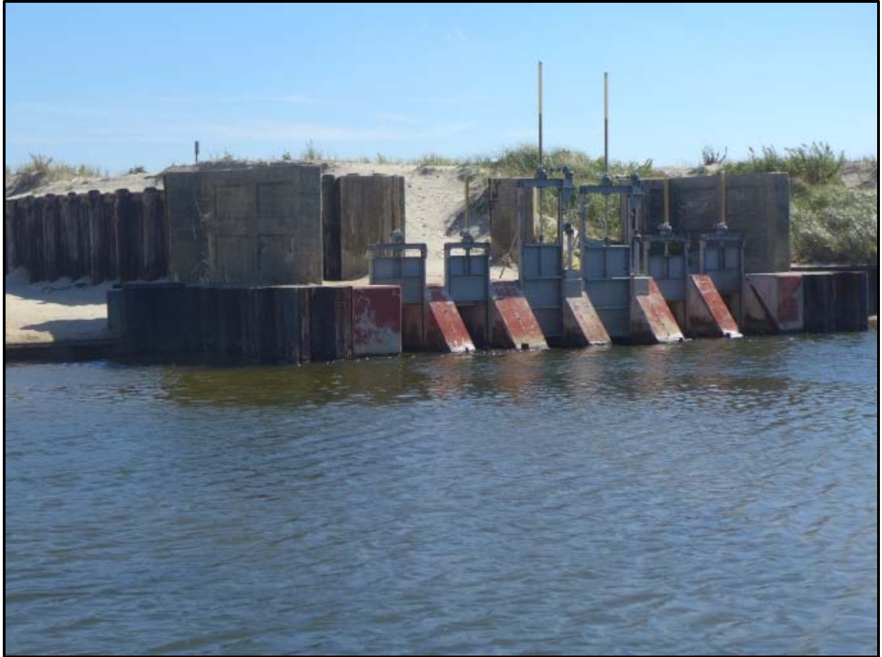
Figure 4: Wreck Pond outfall structure on September 27, 2014.
