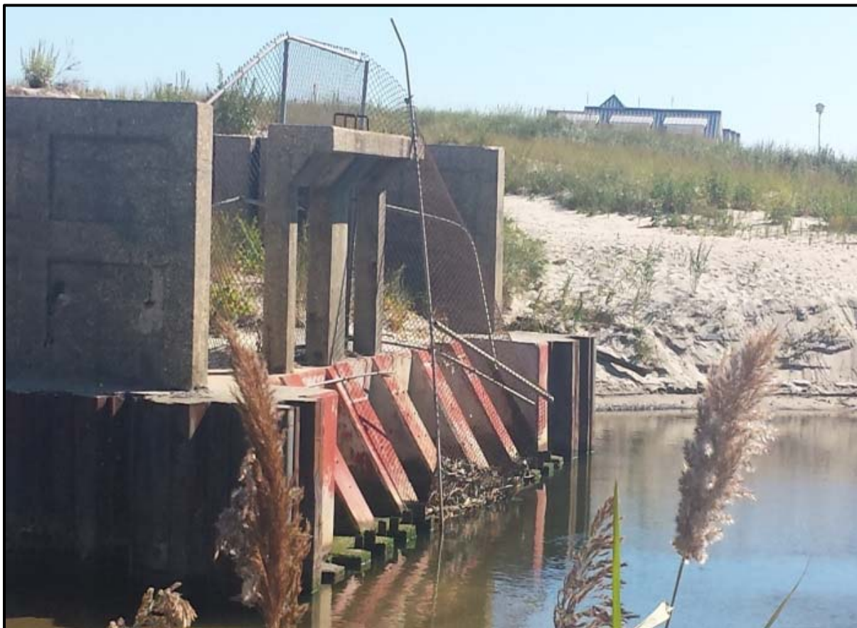
Figure 3: Wreck Pond outfall structure on September 9, 2013.
