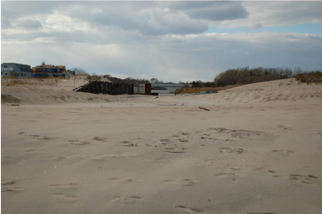
Photo C. Existing emergency spillway and location of proposed pipe (11/08/2013).
