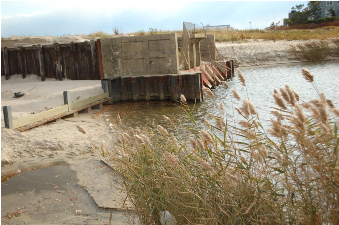
Photo A. Existing outfall pipe and location of proposed pipe (11/08/2013).
