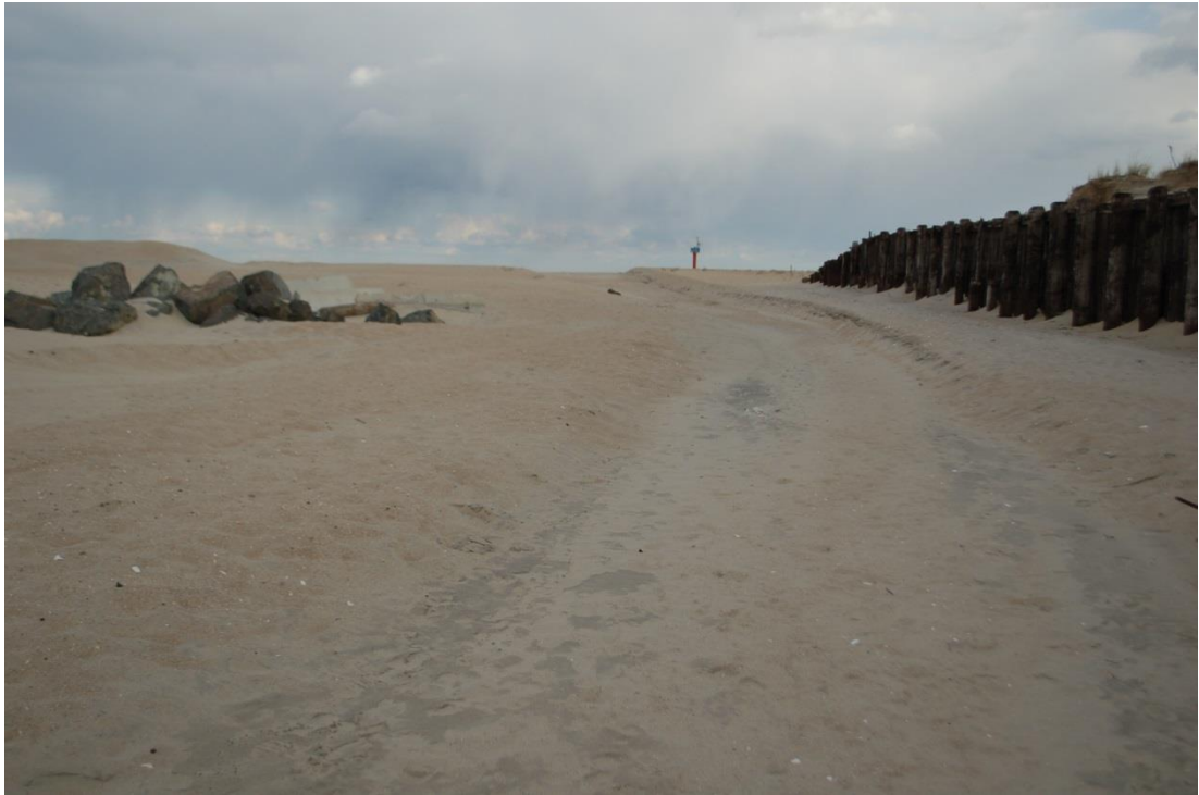
Photo B. Existing emergency spillway and location of proposed pipe (11/08/2013).
