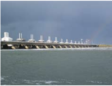
The Eastern Scheldt Barrier protects residents of the Netherlands' Zeeland Province from North Sea storm surges. The barrier consists of gates that are only closed during extreme high tides allowing water to continue to flow through the tidal inlet. (Photo by Amy Shallcross)
