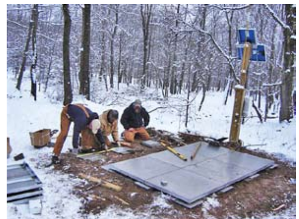
Members of the NYCDEP Watershed Monitoring and Operations Support staff install the first automated snowpack water equivalent monitor (or "snow pillow") in the Neversink Watershed in January 2008. (Photo courtesy of NYCDEP)
