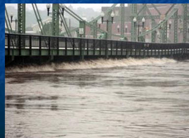
Easton-Phillipsburg Bridge: June 2006
