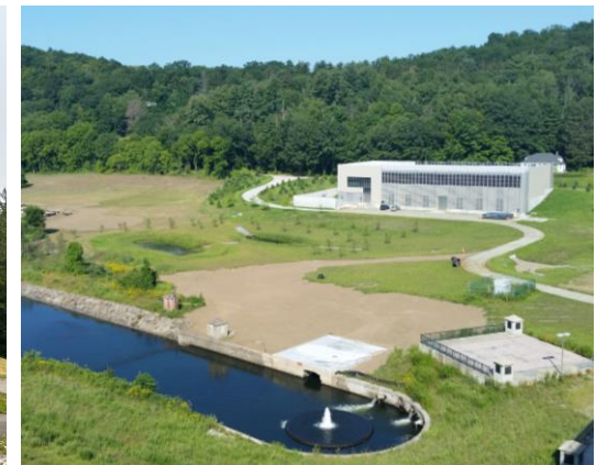
Croton Falls Pump Station
