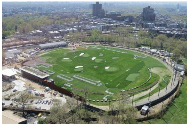
Croton Filtration Plant
