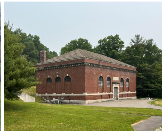
Cross River Pump Station
