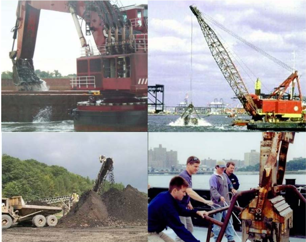
Figure 3.2: Photographs of Dredging Operations
