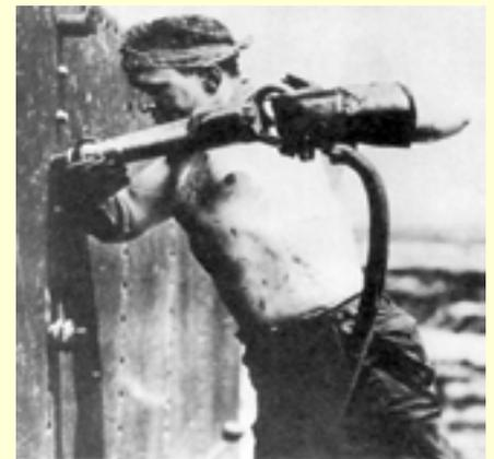
*Riveter at Hog Island Shipyard helping to build the "bridge of ships."*
