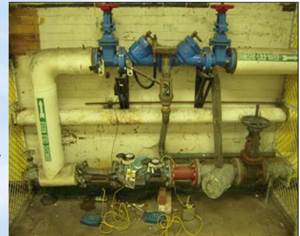
Data-loggers installer on a 4-inch compound meter in a high school
