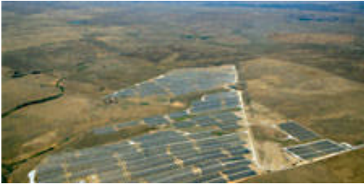
Trujillo Power Plant La Magascona, Trujillo, Spain - 23 MW
