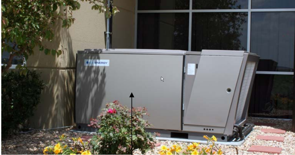
Picture of an Ice Bear 30 unit installed on an office building
