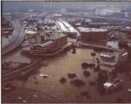
▲ Photo: Harris County Flood Control District, Houston, Texas
