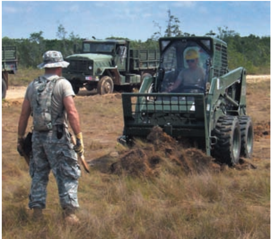
Soldiers from the 110th Engineers Utilities Detachment prepare an area for tents during Operation Tradewinds-Belize. Photo courtesy 110EUD.
