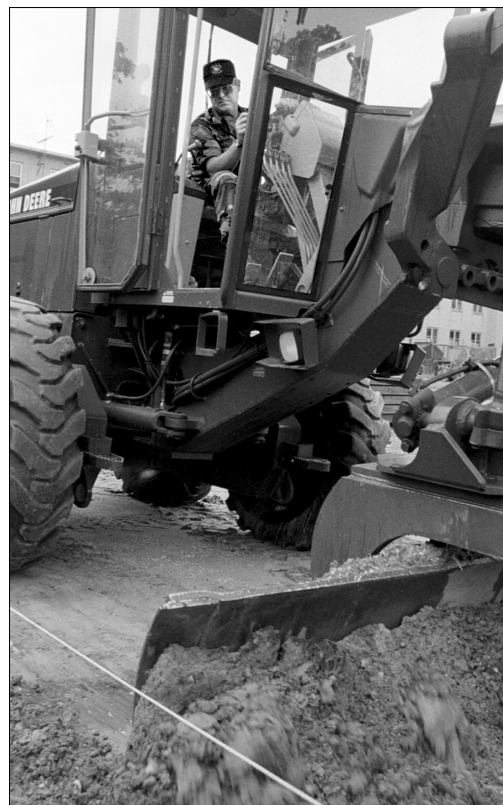
Chief Master Sgt. Herbert Mimler evens out a rough patch in the parking lot addition behind Veterans Haven.
