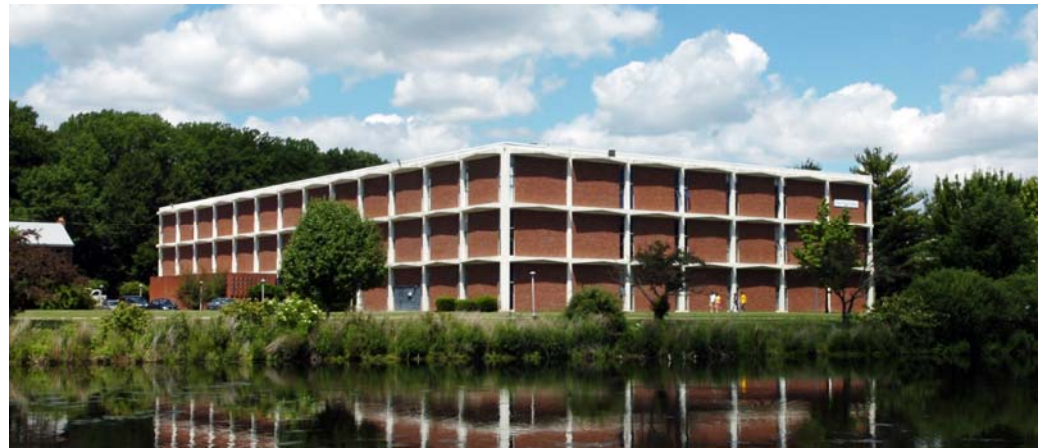
Rider University Tri-Generation Facility
