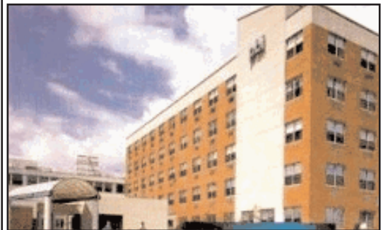
The Authority helped facilitate Passaic Beth Isreal's move from this building, freeing the property for three new schools and an athletic field.
